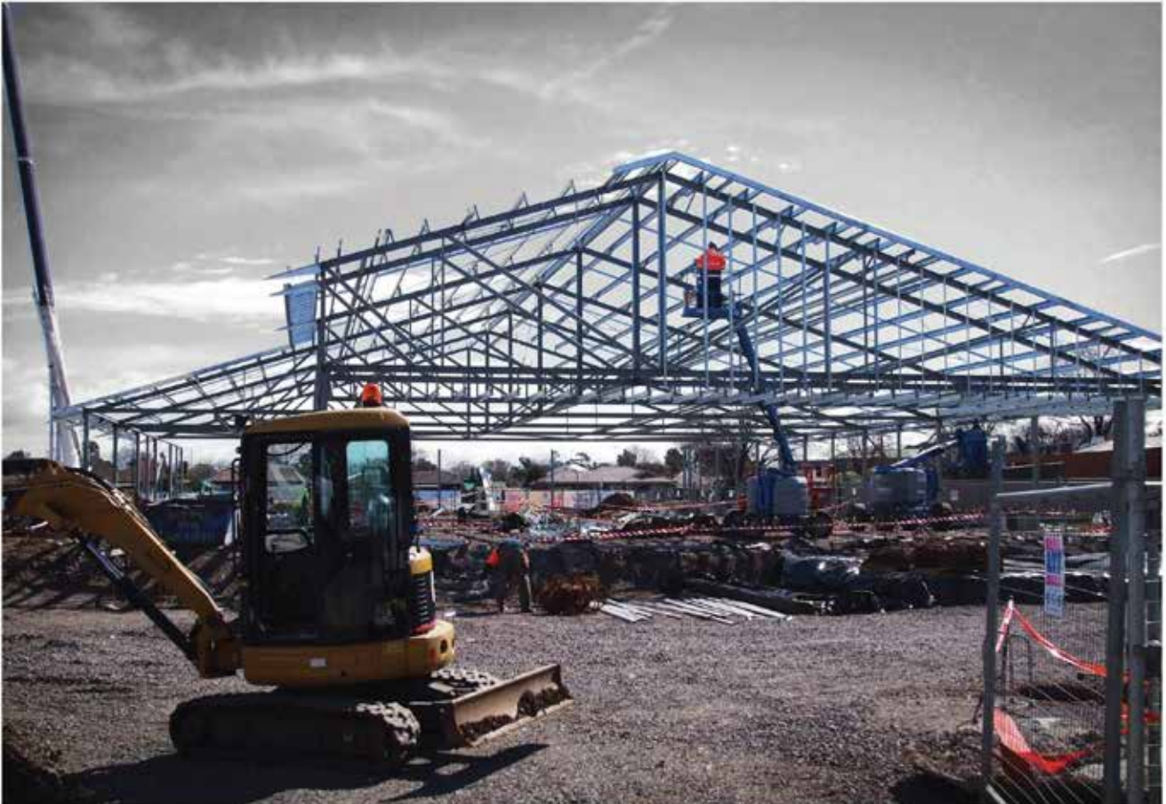
Construction of new Aldi Supermarket in Alfredton
